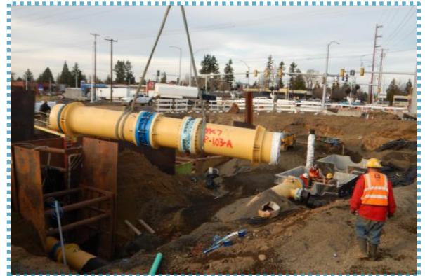
Willamette Water Supply pipeline construction through South Hillsboro continues.
