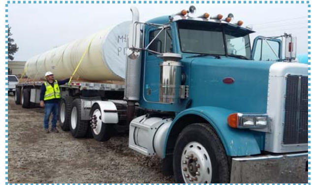
A 66-inch diameter piece of pipe sits on a truck waiting to be unloaded and installed at a Willamette Water Supply System construction site.
