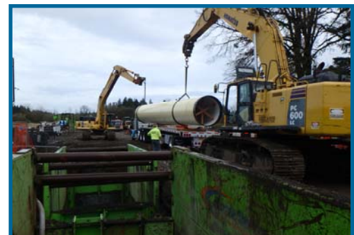
Installation of pipe at the Kinsman Road Partnership Project
